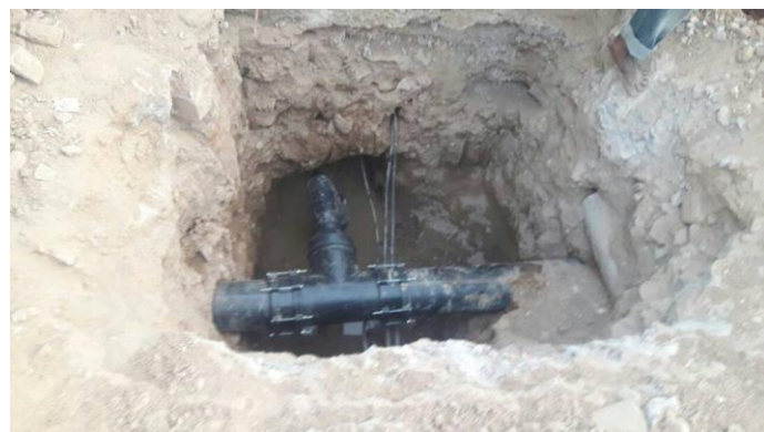
Arresting of water leakage at Acharam Kotala.
