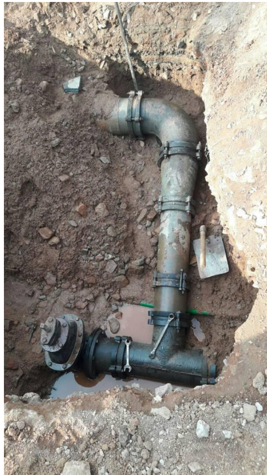
Arresting of leakage in 16 th ward
