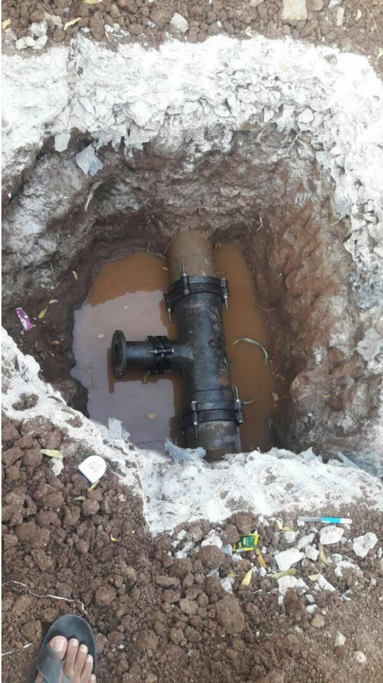
Arresting of leakage at Travelers Bungalow road.
